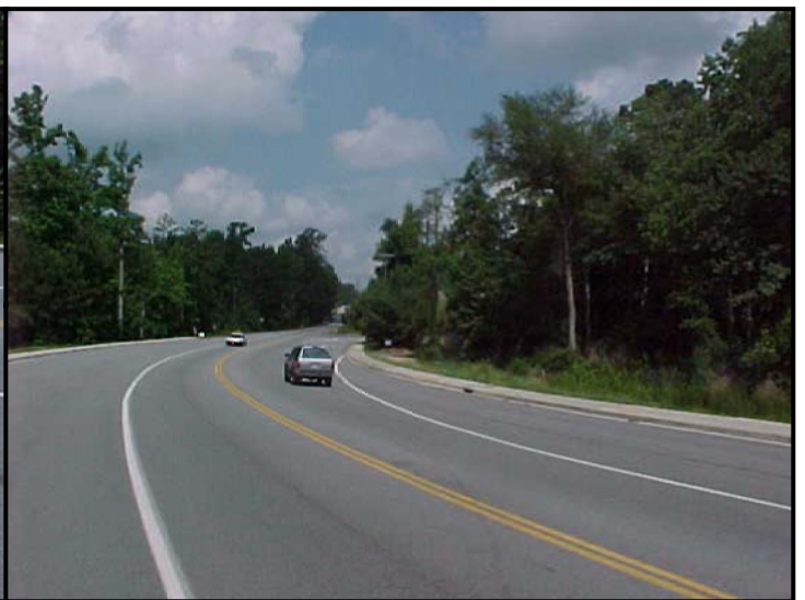
Looking west on Clemson Road
